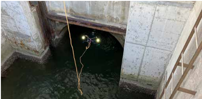
Figure 6: Survey in a confined sewage pump station
