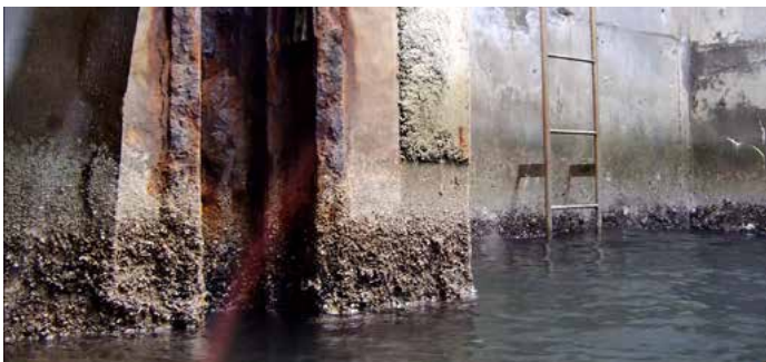
Figure 7: Imaging interior of a pump station
