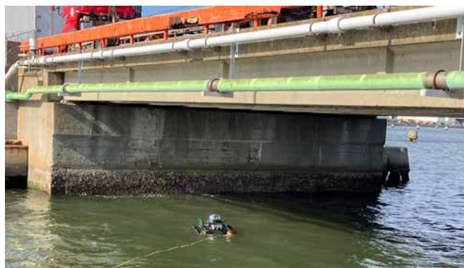
Figure 4: Bridge inspection using a waterproof gimbal camera
