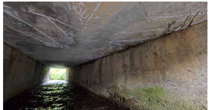
Figure 14: Imaging interior of a culvert using a gimbal camera
