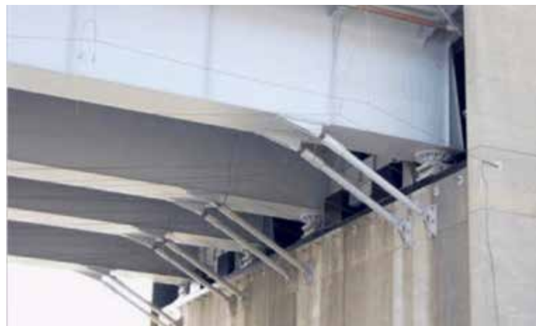
Figure 4: FVDs implantation to reduce responses in bridges by Taylor Devices [17]
