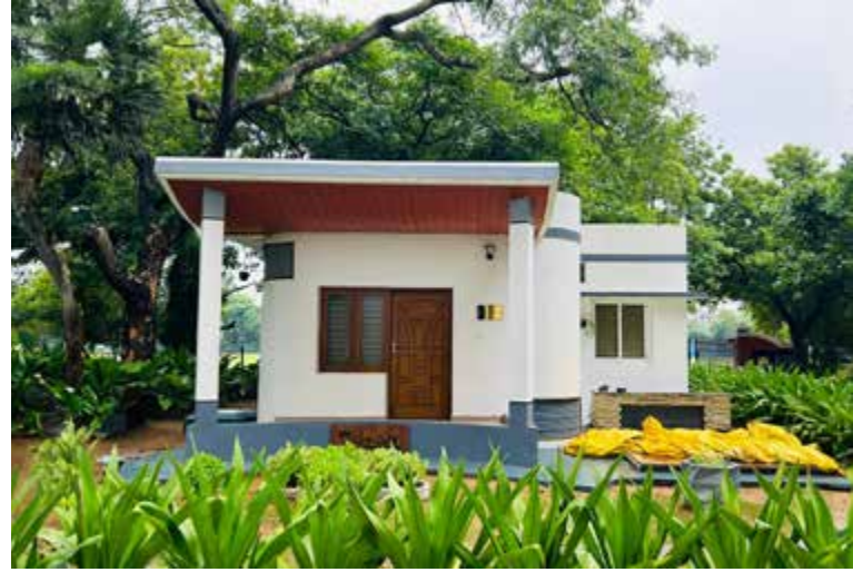
Figure 1: First 3D-printed residential unit in India
