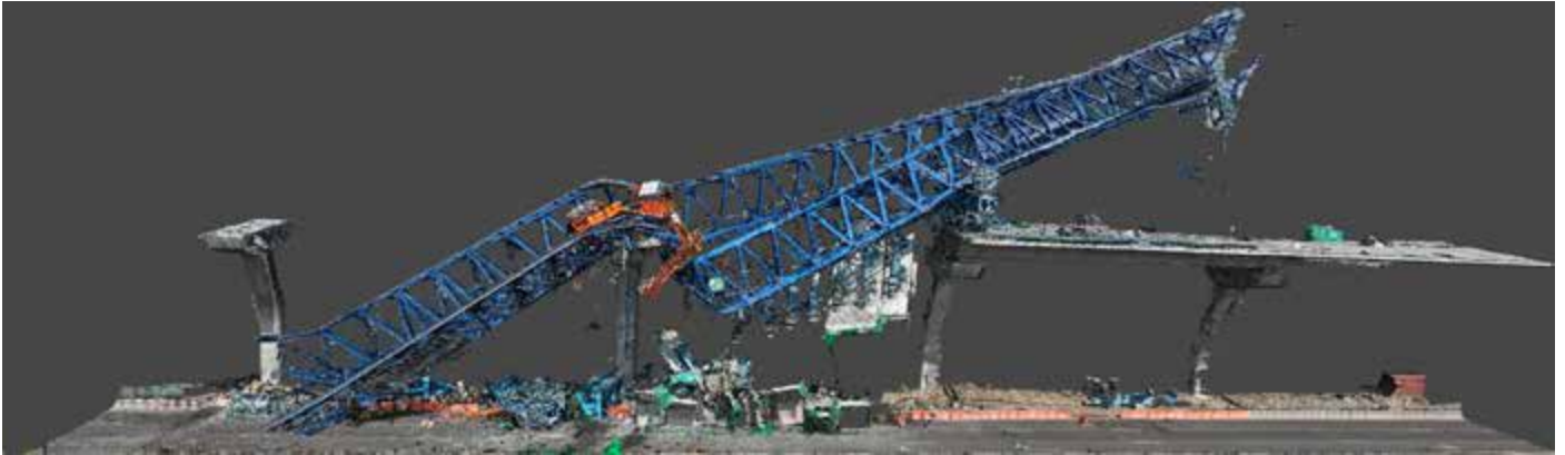
Figure 5: UAV-based 3D reconstruction of a collapsed launching gantry.
