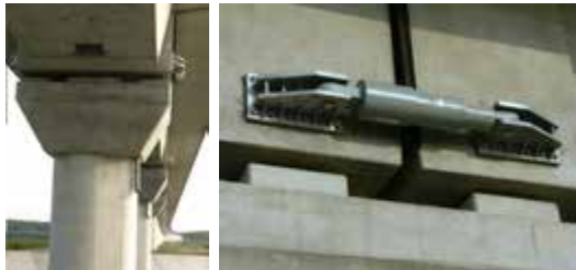
Figure 3: Fluid Viscous Dampers were used for a new bridge section in the Taiwan High Speed Rail system, completed in 2003 [17]
