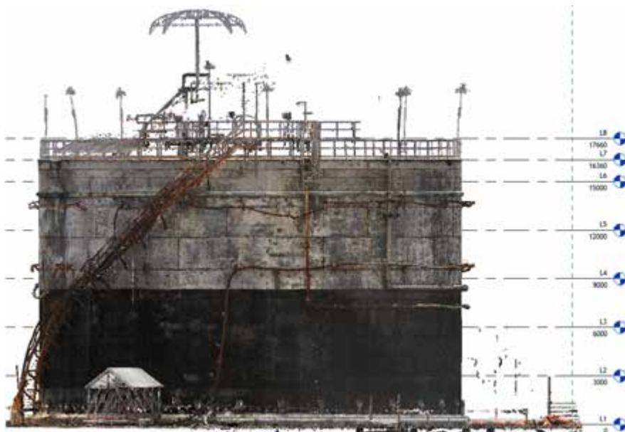
Figure 9: 3D point cloud of a hydrocarbon storage tank.
