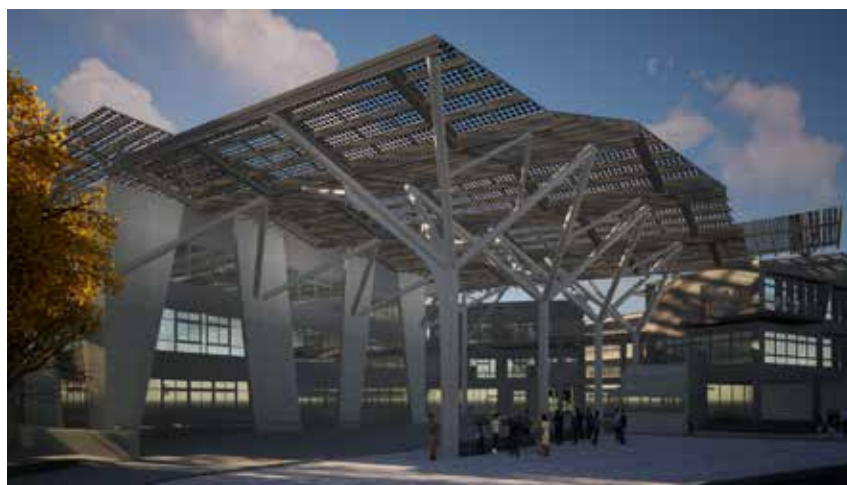
Figure 4: The entrance plaza covered with photovoltaic panels as part of the design to maximize the coverage area
