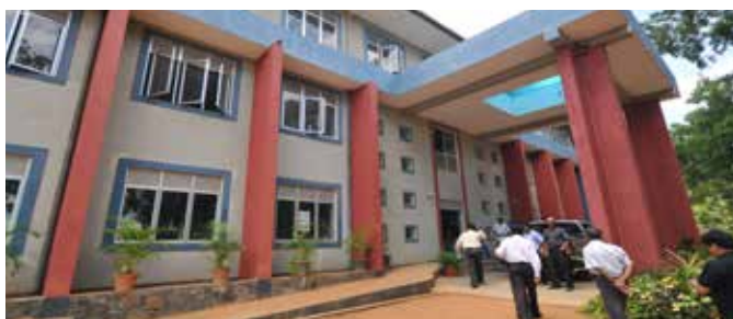
Hambanthota, Sri Lanka: H/Vihargala School was one of the five schools inspected for ADB
