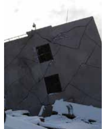
Figure 4 A caved-in building constructed as it is for the training of search and rescue personnel. One and a half floors of the building are below ground, as if caved in following an earthquake. This makes the search and rescue training life-like.
