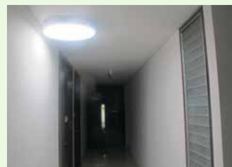
After installation of light pipe
