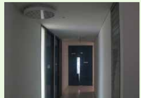
Before installation of light pipe
