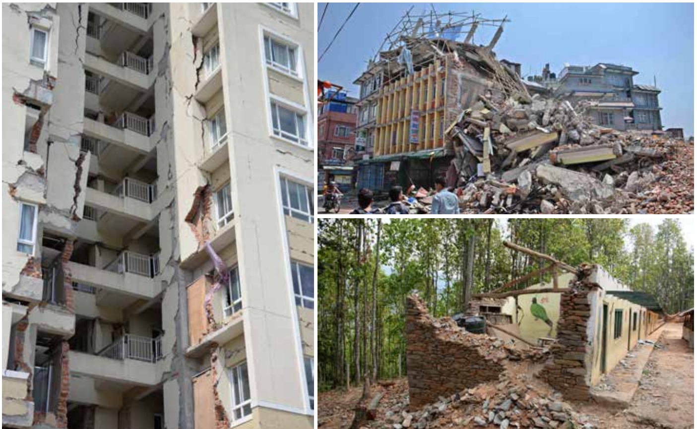
Figure 2: Damages due to Nepal Earthquake in April 2015
