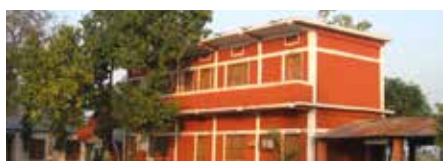
One of the school buildings being retrofitted in Nepal
