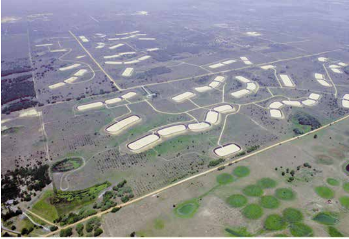
Figure 6: Rapid infiltration basins, Orlando, Florida, United States (Credit: U.S. Geological Survey)
