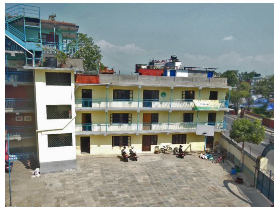
Figure 11: A school building in Kathmandu shows different response. The building originally was load bearing masonry retrofitted with concrete jacket and was undamaged and was available to continue classes after earthquake.
