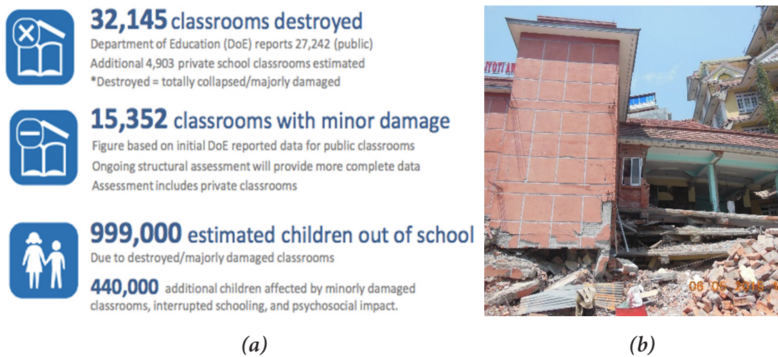
Figure 1: (a) Survey data from Education cluster (the coordinating body for humanitarian education activities) showing the approximate estimate of damage in the earthquake (b) Completely damaged Deepjyoti School in Gongabu, Kathmandu lacking proper seismic details.
