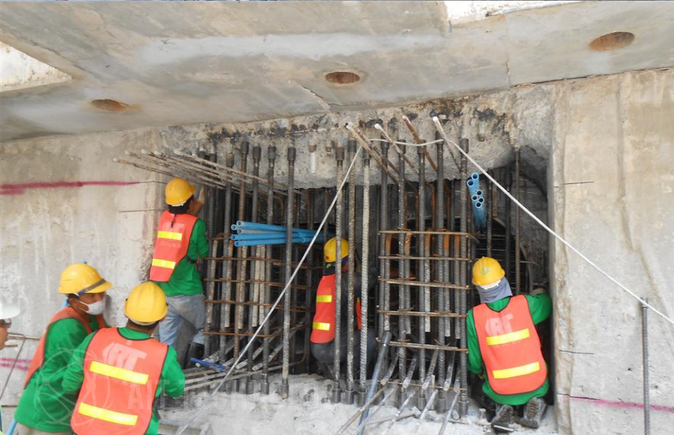
BS12 Sanam Chai Station – Pipe Roofing
