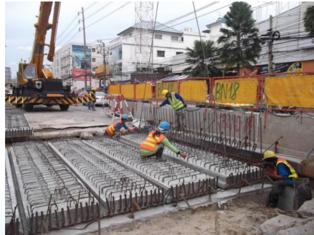
Construction of DSRS Structure at Pier at P-BN10-18 – Zone 1
