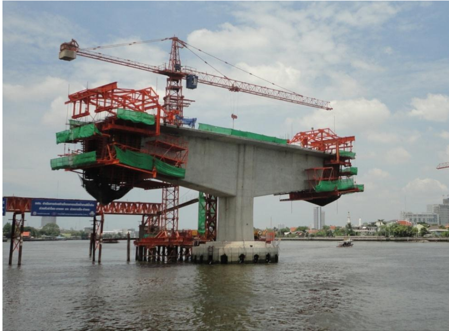
Balance cantilevering construction at P3 (P-BN11-05) Chao Phraya River Crossing
