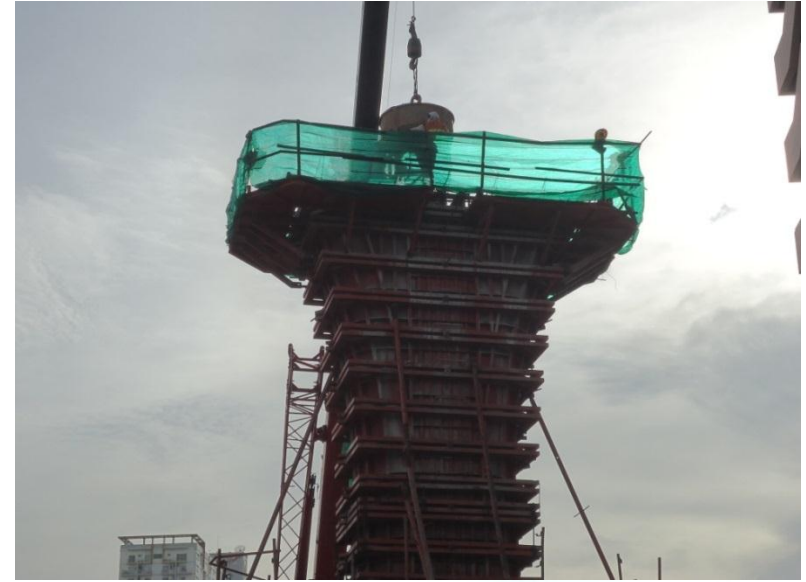
Construction of Pier-head at P-BN11-13 – Zone 2
