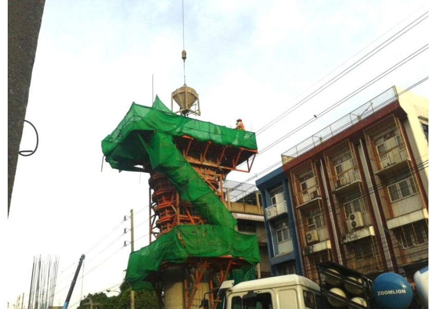
Construction of Pier-head at P-BN10-06 – Zone 1
