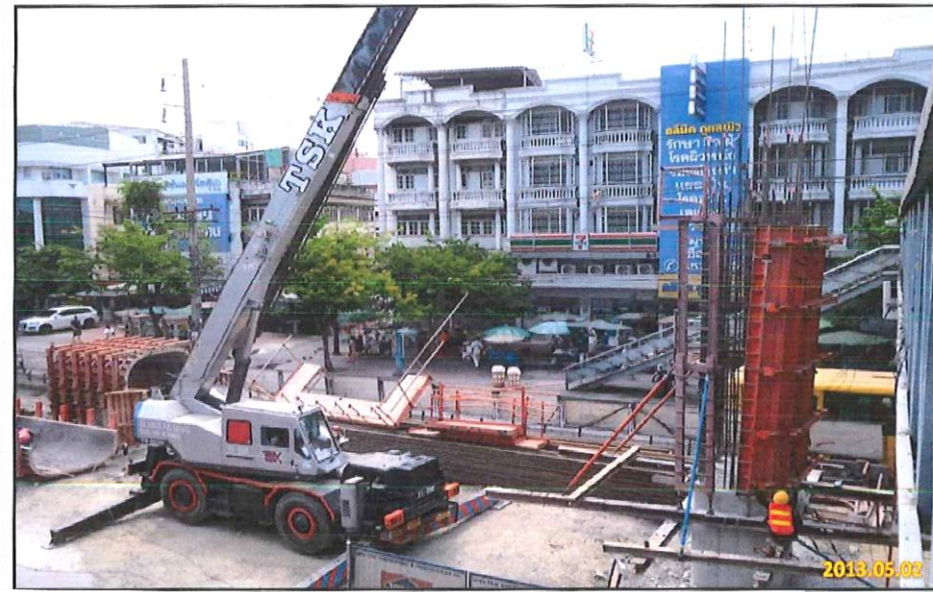
Column Work at P-BS14-28 Phet Kasem Rd.
