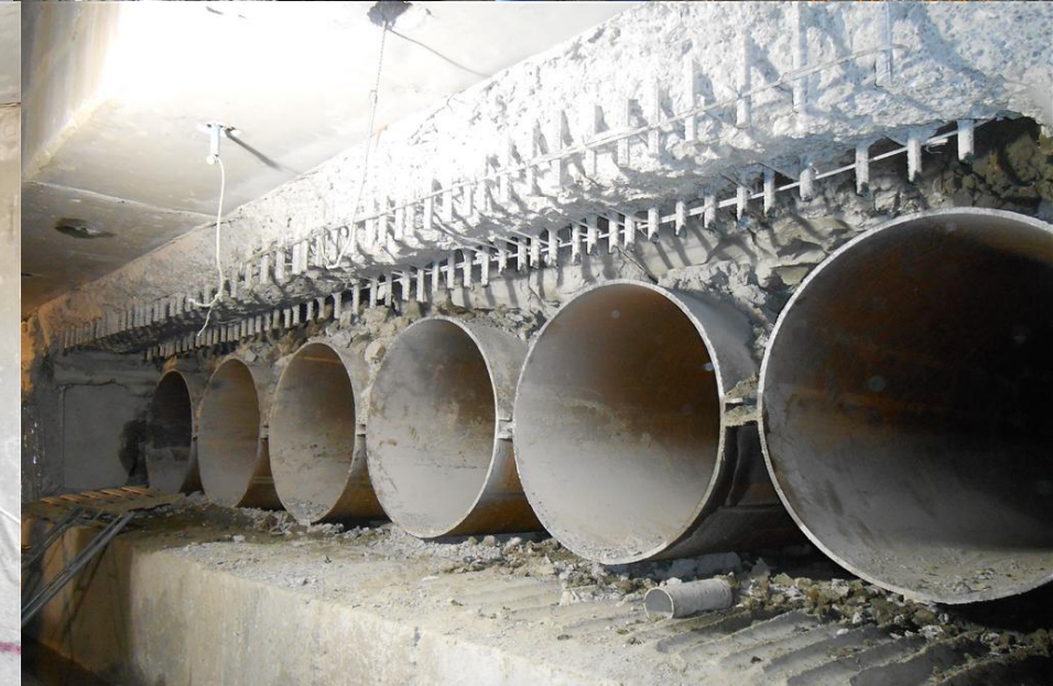
BS12 Sanam Chai Station – Pipe Roofing
