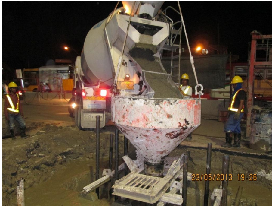
Construction of Barrette Pile (0.80x2.70m) at BN14/2 (L:F) Sirindhorn Station – Zone 3
