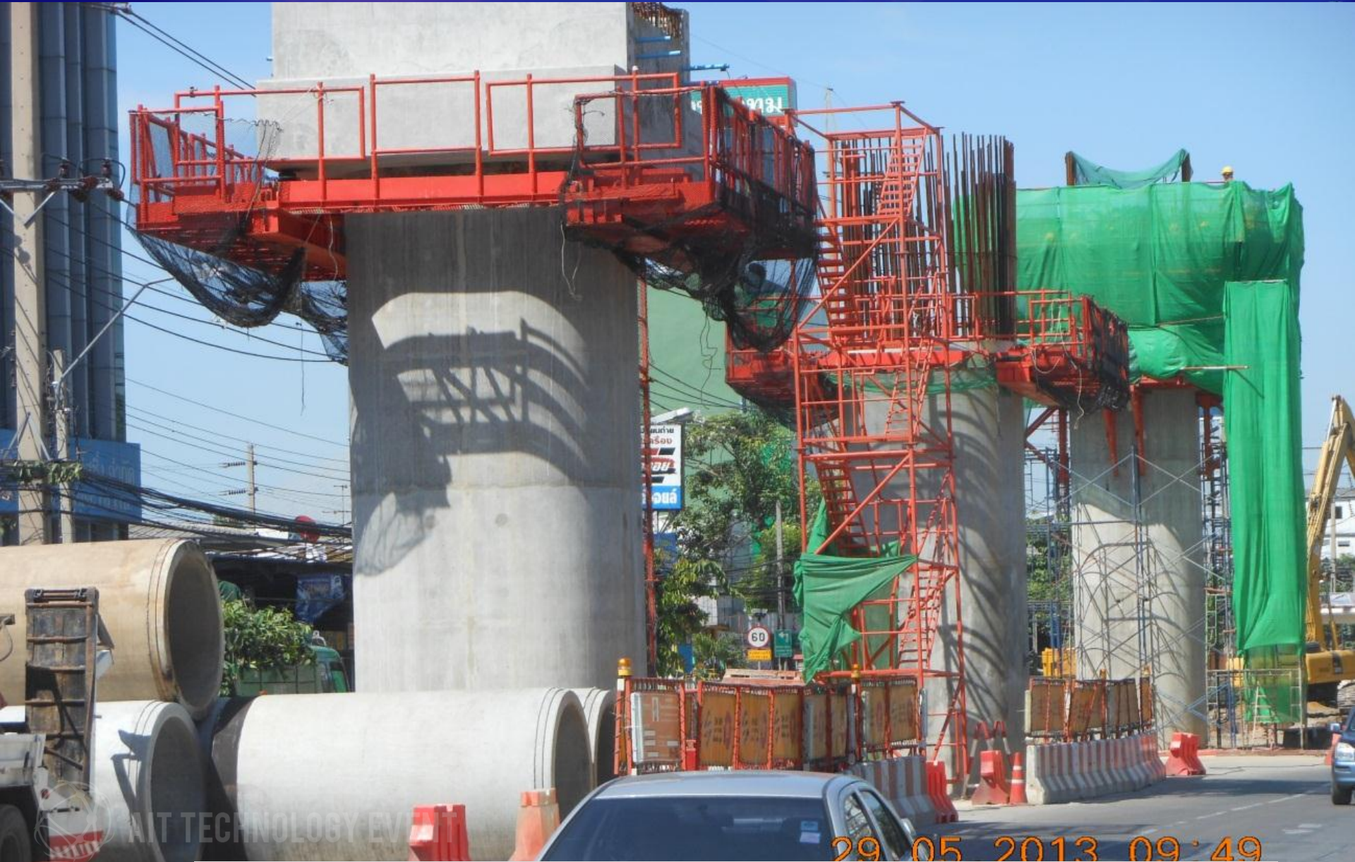
Installation Cross Beam concourse Level Grid Line 4 Bang Phlat Station – Zone 2
