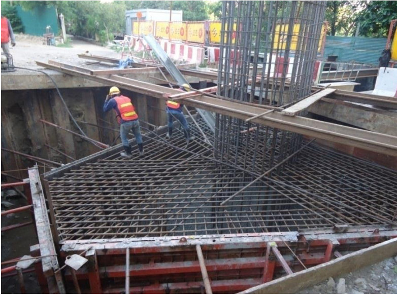
Construction of Pile Cap at P-BN11-12 – Zone 2
