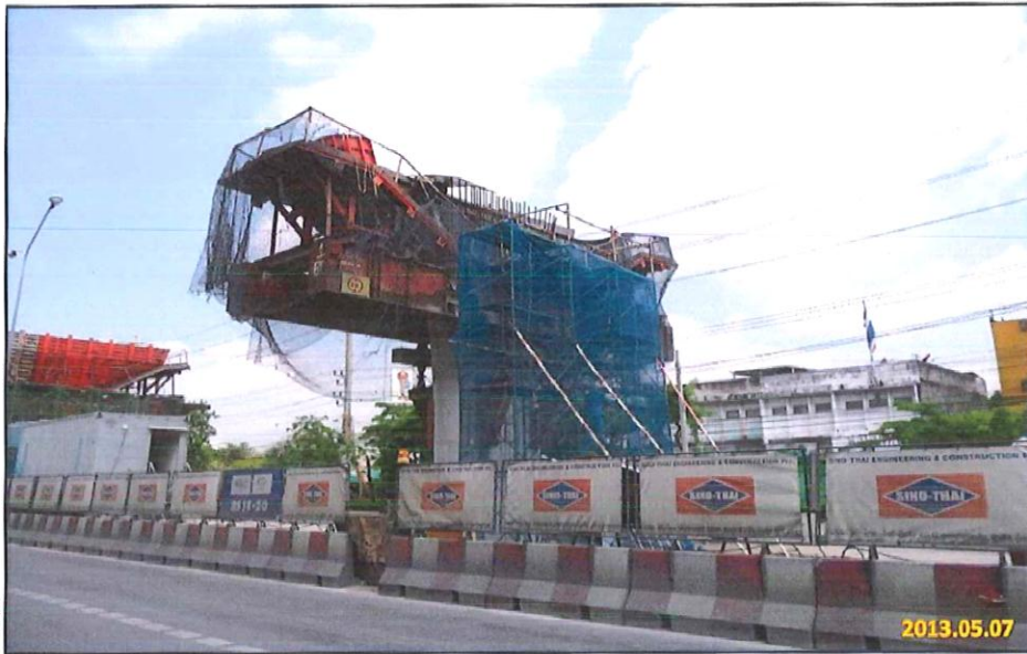
Column Work at P-BS14-20 Phet Kasem Rd.
