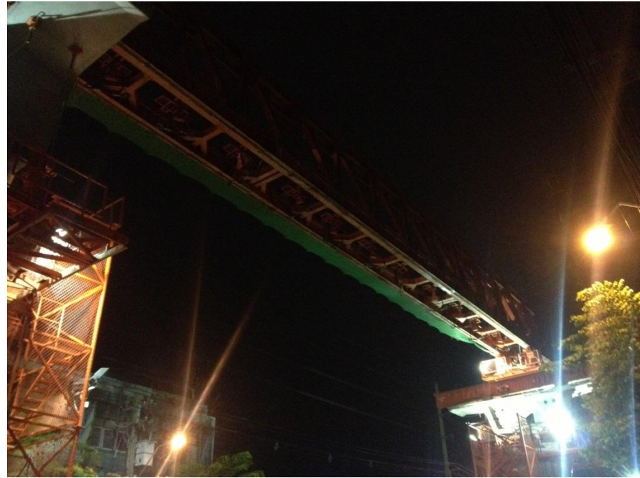
LG2: Erection of Main Truss (Right) at P-BN16-10/P-BN16-09 – Zone 5
