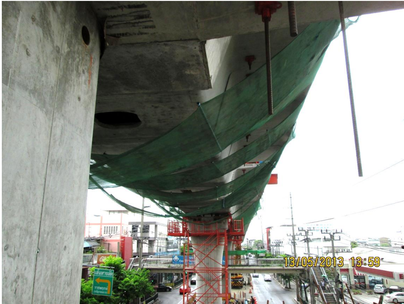
LG1: Segments Erection at Span P-BN17-46 / P-BN18/1 – Zone 5
