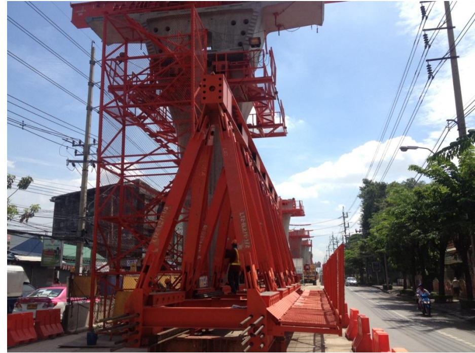
LG2: Assembly Main Truss (Left) at P-BN16-10/P-BN16-09 – Zone 5
