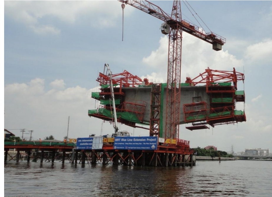
Balance cantilevering construction at P4 (P-BN11-06) Chao Phraya River Crossing
