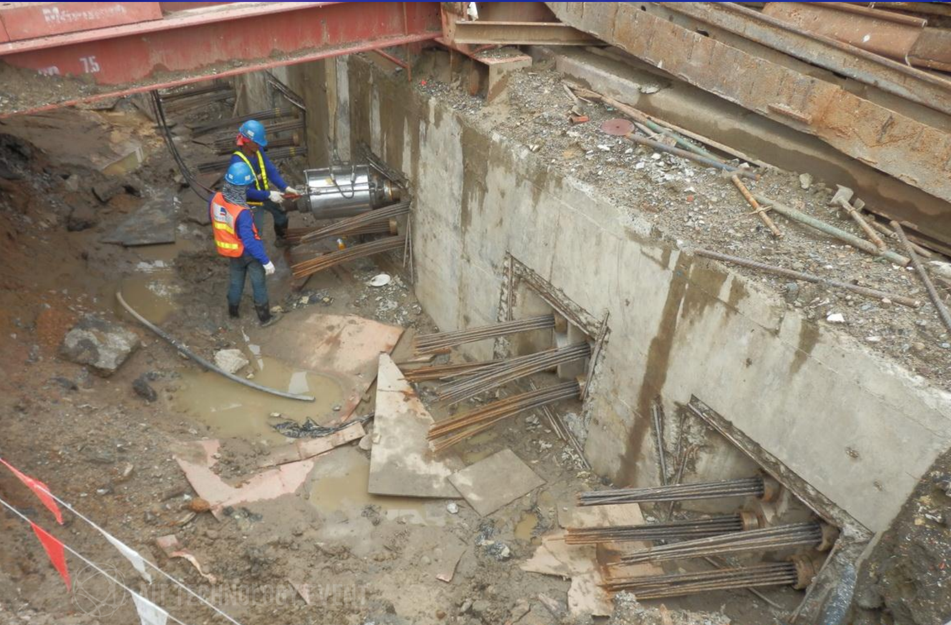
Klong Pradung Krungkasem Construction
