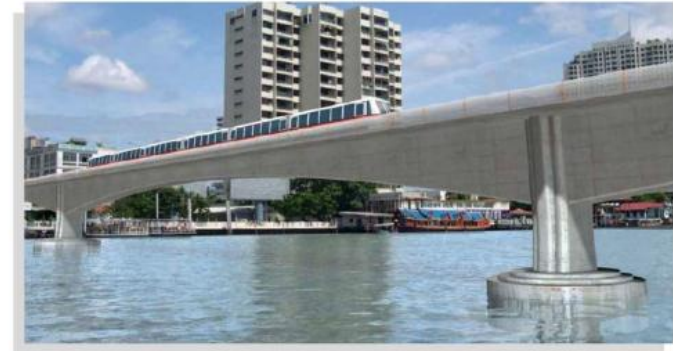
Chao Phraya River Crossing Bridge at Bang Pho
