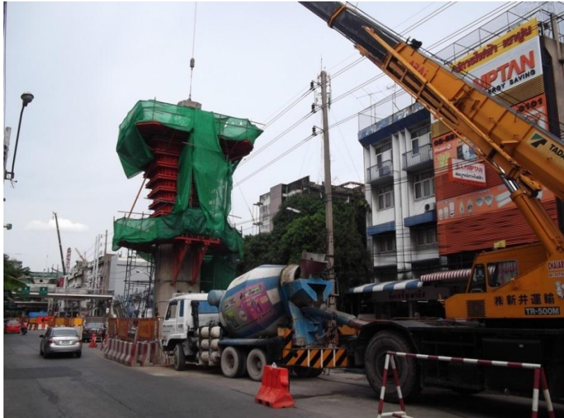
Construction of Pier-head at P-BN10-05 – Zone 1
