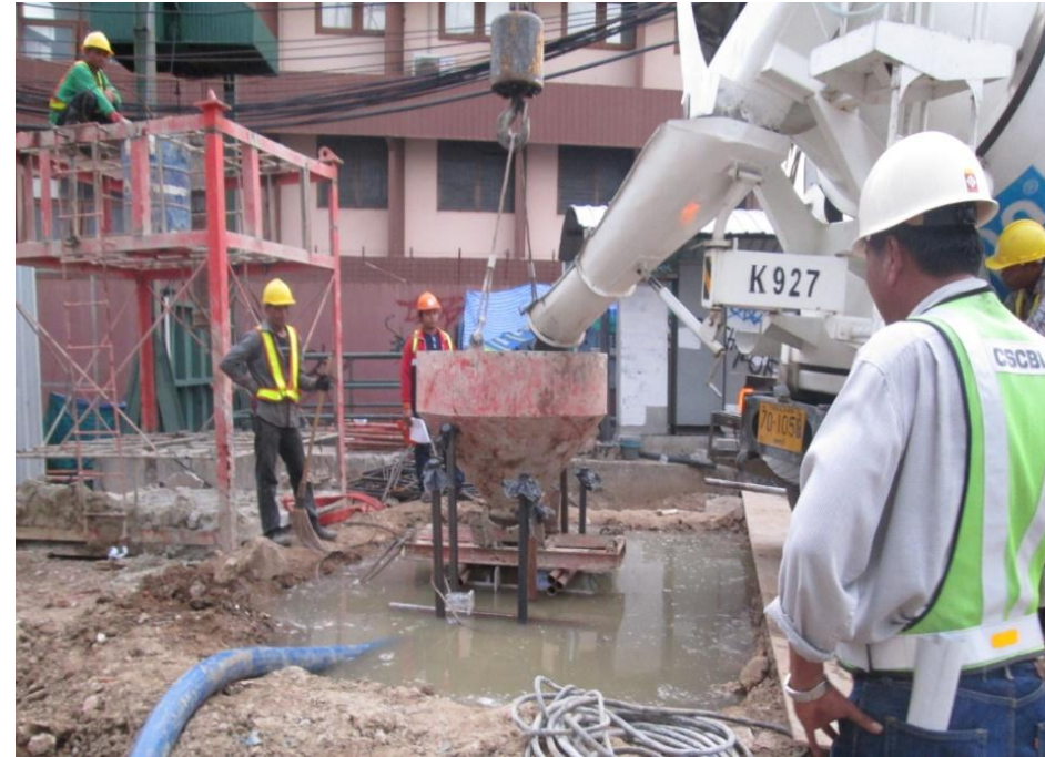
Construction of Barrette Pile (0.80x2.70m) at BN14/4 (L:E) Sirindhorn Station – Zone 3
